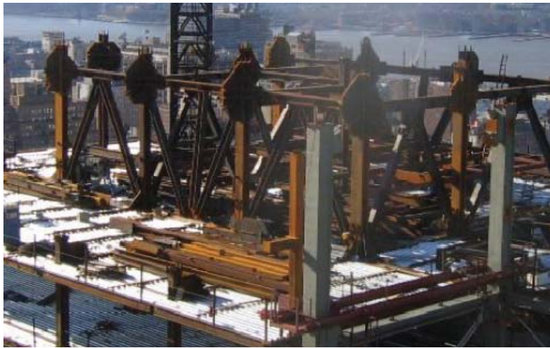
Figure 13: Core bracing during construction, courtesy of Thornton Tomasetti
